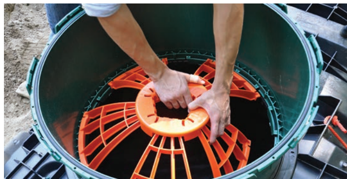
Infiltrator's five arm Safety Star system is equipped with a folding arm for easy installation.
